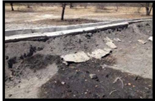
The irrigation canal pictured above was damaged by livestock, rendering the system useless. It is
