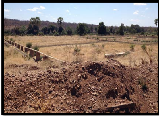
Staffing is critical! Notice the above ground, elevated PVC pipe which leads from a storage dam to supply irrigation canals. PVC pipes deteriorate rapidly when exposed to the elements. The pipe is running down hill and is gravity fed therefore this pipe should have been buried to protect it from the elements, animals and children. The more than 20 cement and brick pillars supporting the pipe were a waste of valuable resources. A lack of checks and balances by the implementer allowed this poor design.
