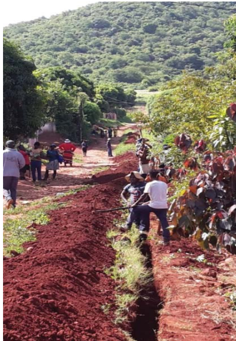
Figure 8 Semi-skilled workers digging trenches in Maswie/Tshakhuma (photo credit Barbara van Koppen)
