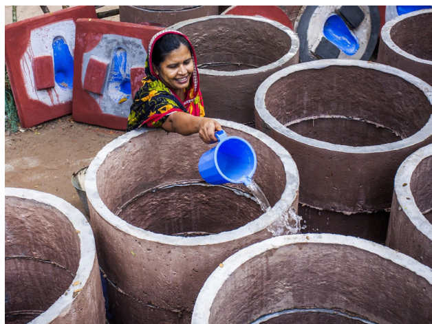
Rings are important to line the pit. Photo credit iDE
