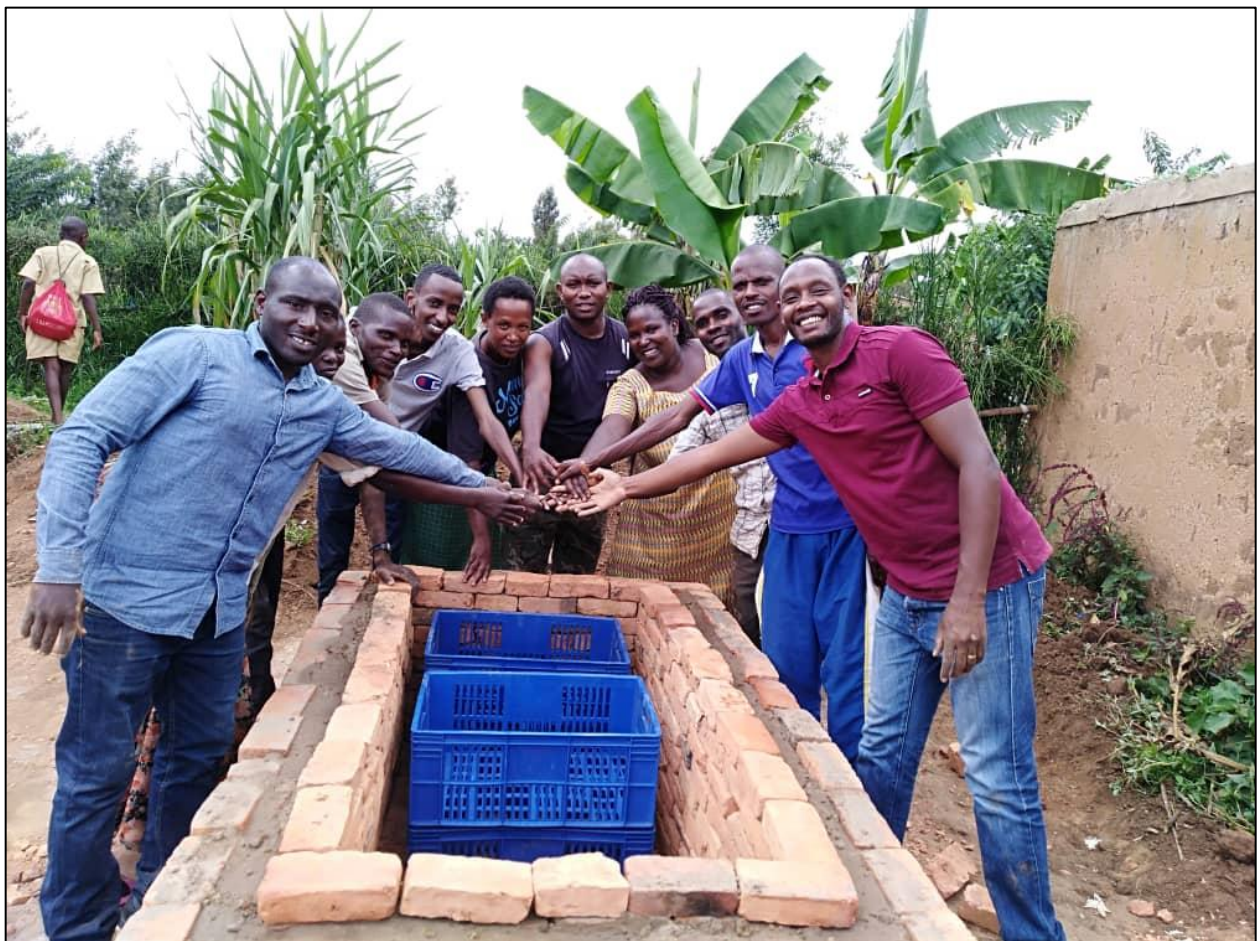
A completed brick Zero Energy Cooling Chamber in Gatisbo, Rwanda.
