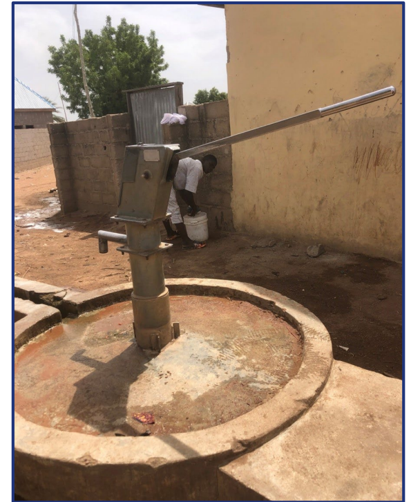
Borehole in Yola South
