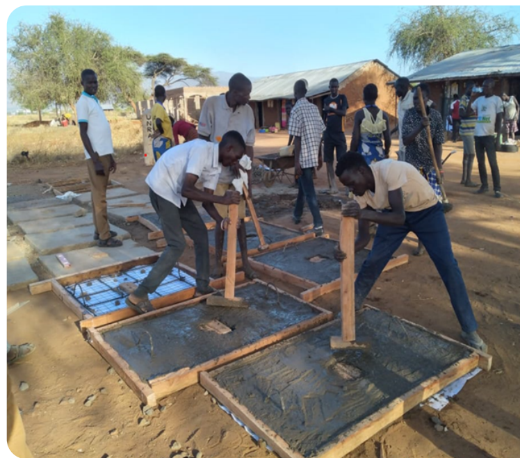
Entrepreneurs learn how to create concrete latrine slabs during training.
