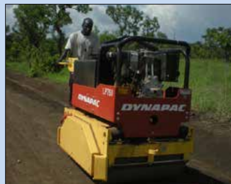
In Uganda, a small roller compactor is used on a road bed.
